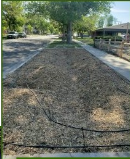
Above: Drains, gravel, soil, mulch, and irrigation lines are installed. Left & Below: Spring of 2020 the City of GJ planted two trees in bioswale, by summer all was thriving.
