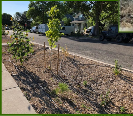
It Works! March 2020, rain runoff flows into freshly dug bioswale on Chipeta Avenue.
