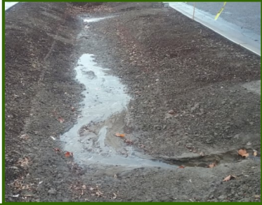
It Works! March 2020, rain runoff flows into freshly dug bioswale on Chipeta Avenue.
